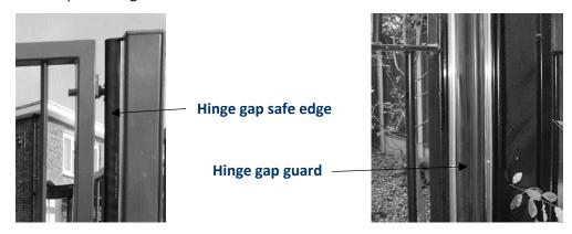
Where a gate creates a <u>shearing</u> hazard as it passes a fixed support element, wall or fence (very common with a sliding gate) there must be rubber safety edges or fencing to prevent access to the dangerous movement. These areas could alternatively be protected with a light curtain.
