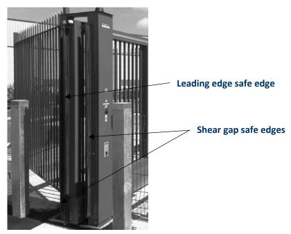
Rather than use additional safety devices, smart design that eliminates changing hinge gaps and use of intelligent drive units can with great care be utilised to provide the required level of safety.
